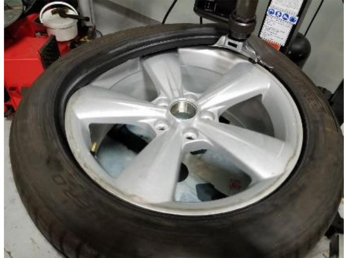
Next, remount top bead and this time use the bar to force the bead into the drop center, Notice how the machine stays in its higher speed now that the load is light.
